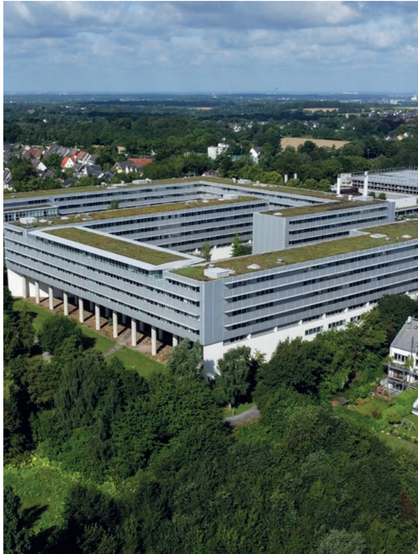
THEODOR-ALTHOFF-STRASSE 39-47 (BÜROPARK BREDENEY)
